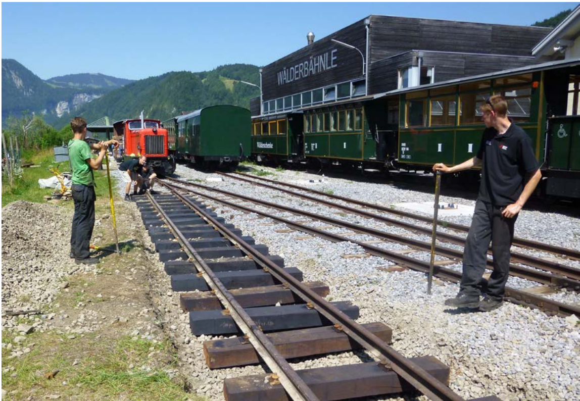
Photograph: Bregenzer Forest Railways-Railway construction-Bezau_20130805-Martin Strohm.jpg
