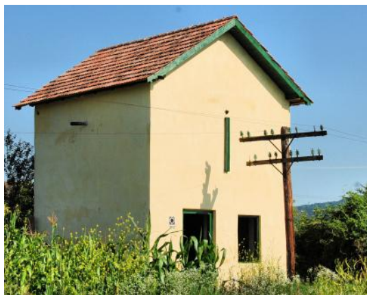
Before and after the restoration of the Cornatel water tower.
